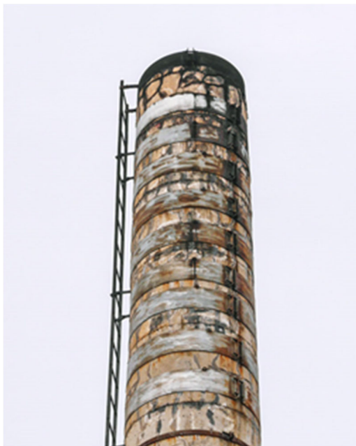
Fig.3 Bathhouse chimney 50-60 years old in need of soot removal by Photographer:deceased Kazunori Miyoshi
